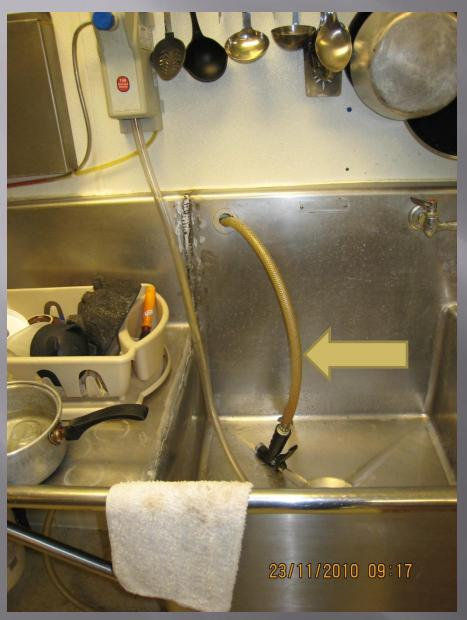
Photo shows spray gun and hose below flood rim of fixture. No device is connected to hose to prevent wastewater from flowing back into drinking water supply.
