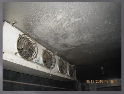
Photo shows fungi growth on fan covers and ceiling of produce walk-cooler. Spores from the fungi can negatively effect food and workers.
